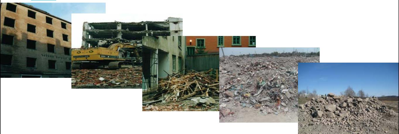
~50% by weight is concrete and masonry
